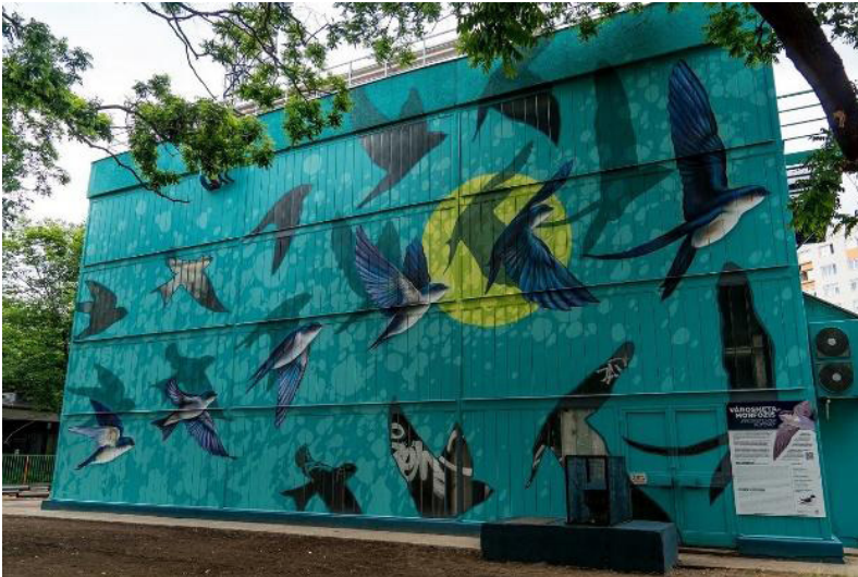
Figure 2: Swallow Nest heating plant
