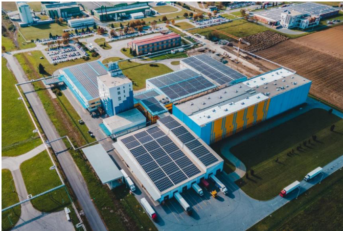
Figure 4: Podravka's rooftop solar plant
