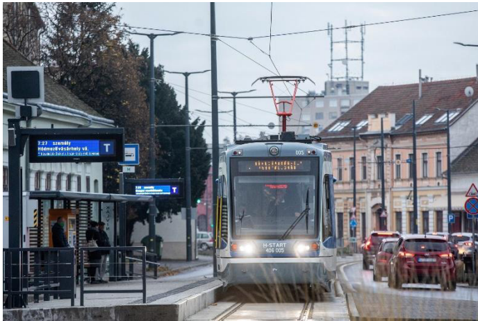
Figure 1: Tram train uses standard city tram tracks
